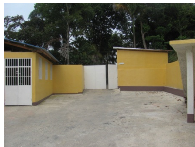
Monastery Front Entrance 1
