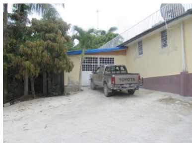
Old Patio now Enclosed 1
