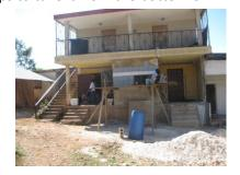
was mounted and the tank was placed on the second floor (also under a roof). We finished up the plumbing and went to hook up the electrical only to find they had lots of electricity, but it was all 220VAC on a European genset which means there was no neutral leg to tap off 120VAC, so we used a
